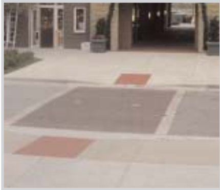
APPROPRIATE PEDESTRIAN CROSSWALK
